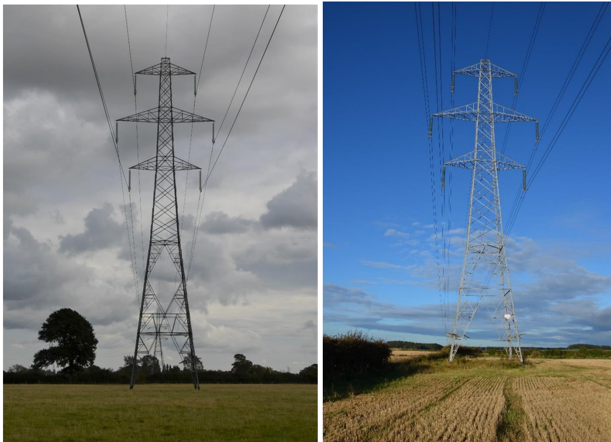
Figure 2.2 - Example of single conductors (left image) and twin conductors (right image)
